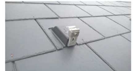
Slate Bracket + Flashing
